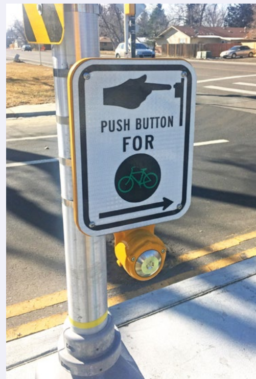
Modification of R10-4 to be applicable to a bicycle signal
