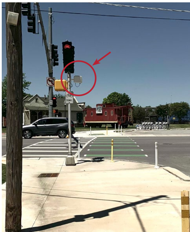
This microwave detector in Huntsville, AL, calls the bicycle signal only for approaching bicyclists who are within the separated bike lane. Microwave detectors can determine if the bicyclist is approaching or moving away from the intersection to avoid false calls.
