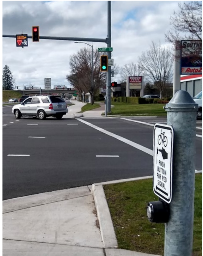
This push button activates a bicycle signal along a separated bike lane in Eugene, OR
