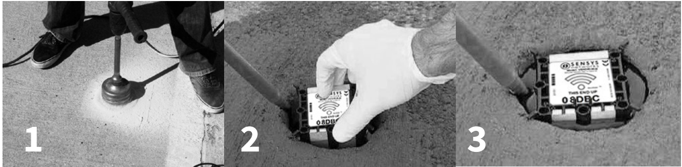
Installation includes (1) coring out a hole in the pavement, (2) placing the sensor, and (3) backfilling with epoxy
