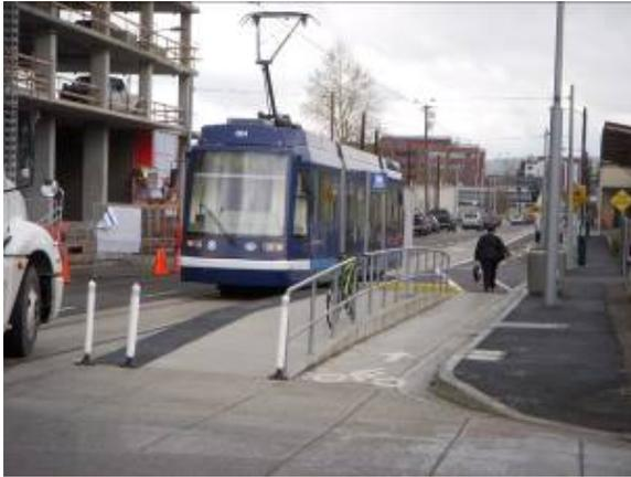
*This detour design in Portland, on a flat grade with a grade separation between cyclist and pedestrian zones, has been well-received to date.*
