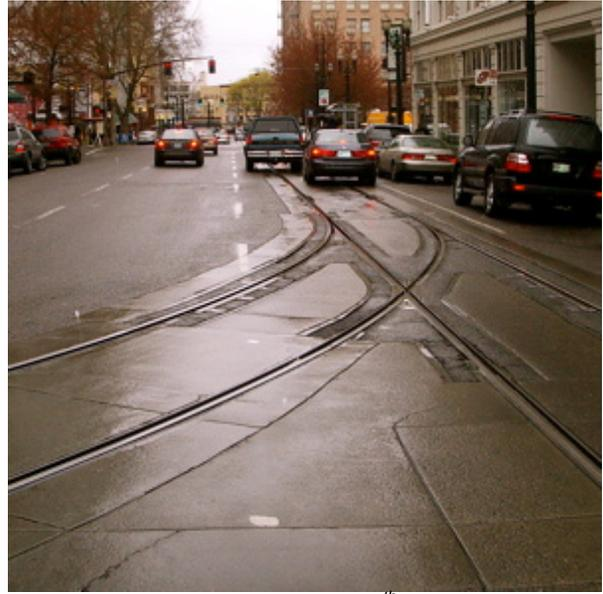
*Track Curves in Portland on SW 10<sup>th</sup> between Morrison and Alder: In order for a streetcar to turn it must create a wide angle. The resulting geometry can be difficult for cyclists to cross. The situation becomes more dangerous when the tracks are wet because they are slick and require a crossing angle closer to 90°.*
