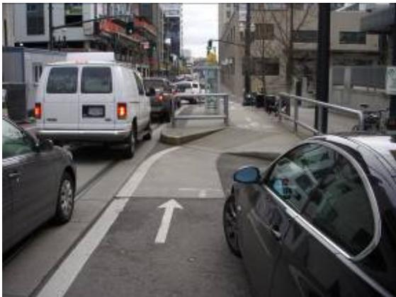
*This sidewalk detour around a transit stop in NW Portland successfully eliminated the “pinch point” danger as the curb extension joins the tracks, but has been a source of conflict for cyclists and pedestrians (perhaps due to a slight downhill grade that increases cyclist speed).*
