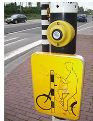
*A button-actuated countdown bicycle signal head creates a separate signal phase for bicycles to eliminate tram conflicts in Amsterdam.*
