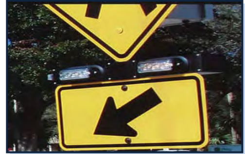
Rectangular Rapid Flashing Beacons are installed between the crossing sign and the supplemental arrow. Source: FHWA.
