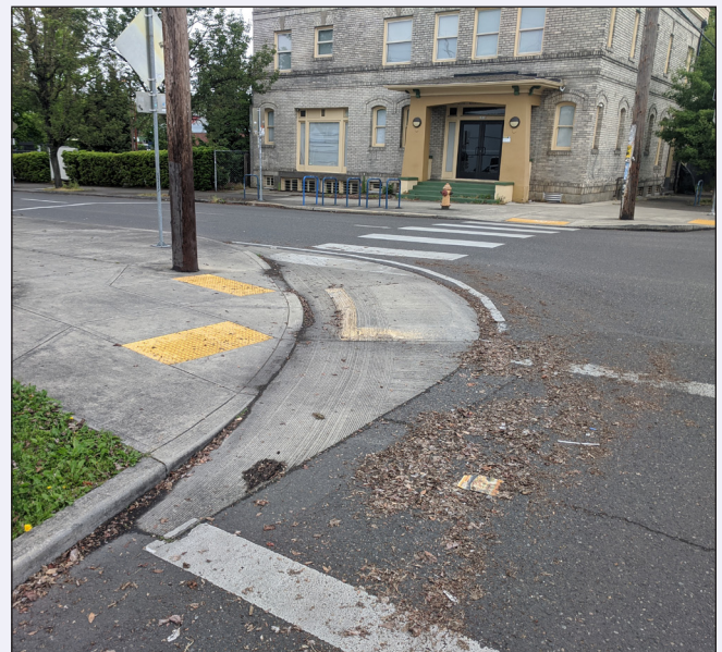
ABOVE LEFT: A corner “wedge” at the intersection of two one-way streets in downtown Portland. ABOVE RIGHT: A concrete corner speed hump as a right turn treatment. Part of the center area of the apron is raised as a deterrent to passenger vehicles. BELOW: A second example of a concrete corner speed hump, with a more pronounced “hump” area.
