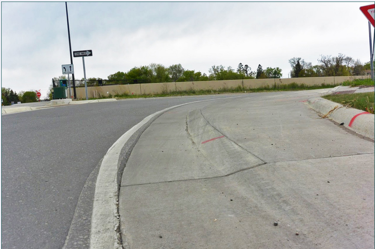
ABOVE: A road user's view of one of the right turn channels at the interchange with a traversable apron treatment. BELOW: A close-up view of the same channel showing the traversable curb profile.
