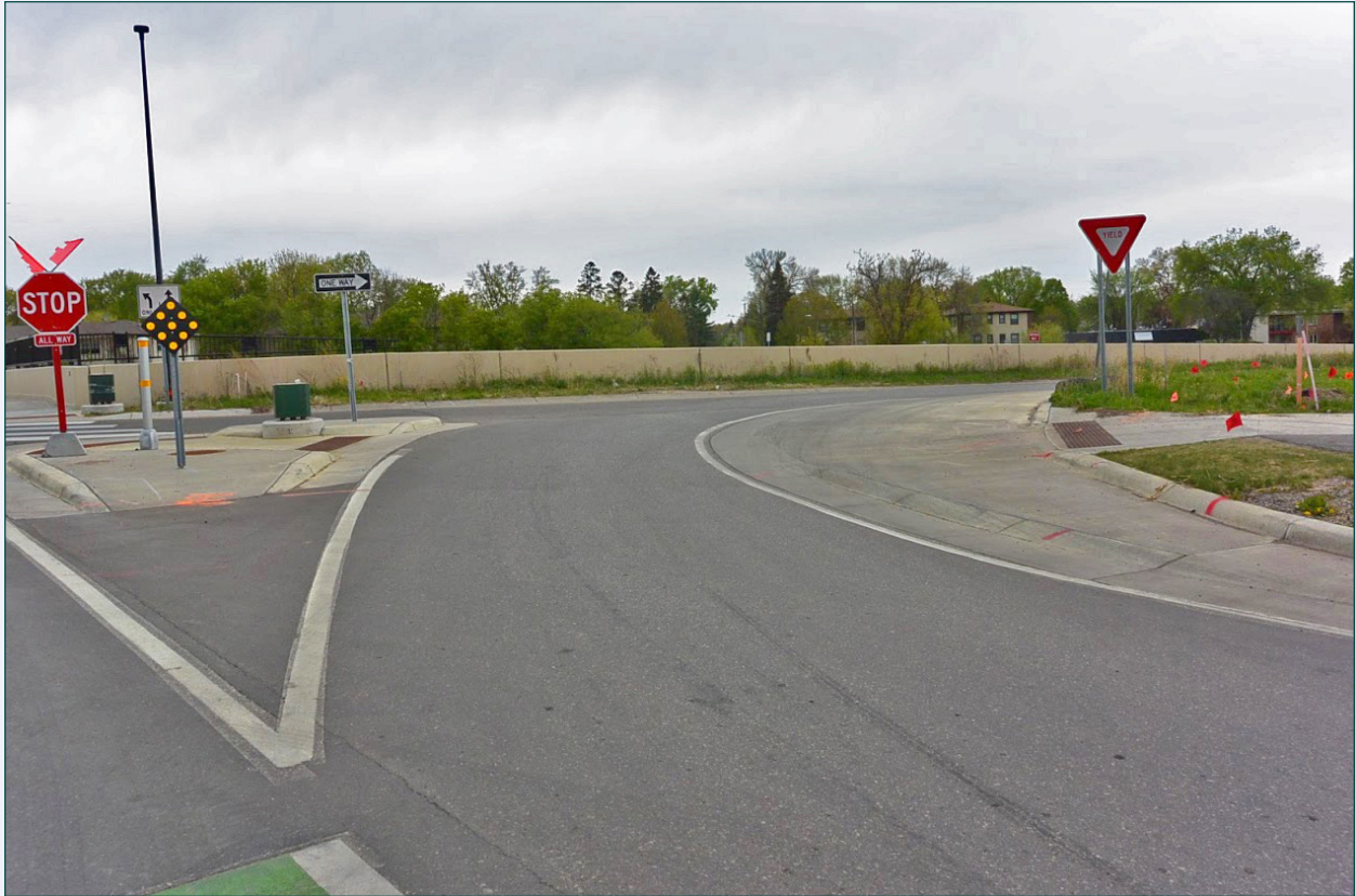
ABOVE: A road user's view of one of the right turn channels at the interchange with a traversable apron treatment. BELOW: A close-up view of the same channel showing the traversable curb profile.
