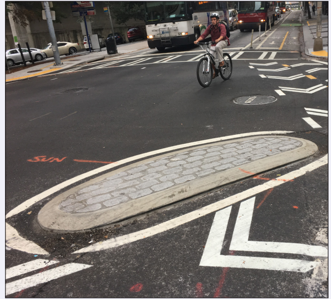
ABOVE LEFT: The corner design treatment applied at 10th NW and Brady. The apron is defined by a mountable curb with a significant vertical component. ABOVE RIGHT: The corner design at Peachtree Center and John Portman. BELOW: Two bicyclists queuing behind the mountable corner apron at Peachtree Center and John Portman.
