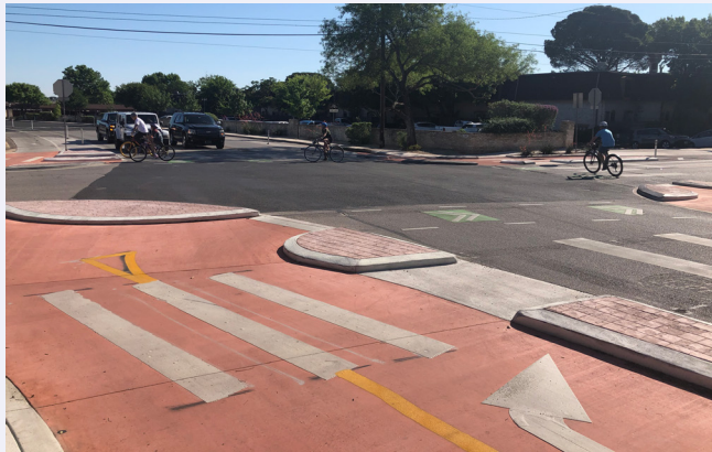
A more recent implementation of a protected intersection corner that is mountable only to fire trucks. The color helps distinguish this corner to other drivers so as not to hit it.
