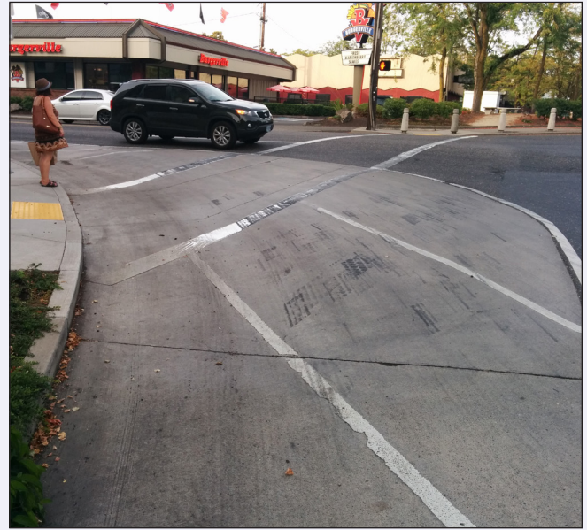
ABOVE LEFT: A corner “wedge” at the intersection of two one-way streets in downtown Portland. ABOVE RIGHT: A concrete corner speed hump as a right turn treatment. Part of the center area of the apron is raised as a deterrent to passenger vehicles. BELOW: A second example of a concrete corner speed hump, with a more pronounced “hump” area.
