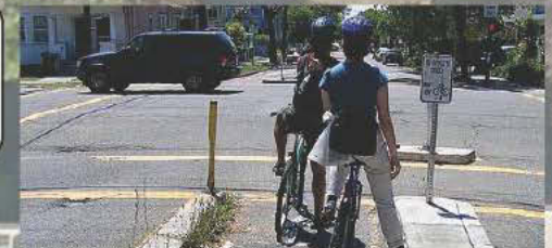
A protected through bicycle lane provides a waiting space for bicyclists at this intersection while also managing through vehicular traffic volumes along this route by forcing vehicles to make a right turn only.
