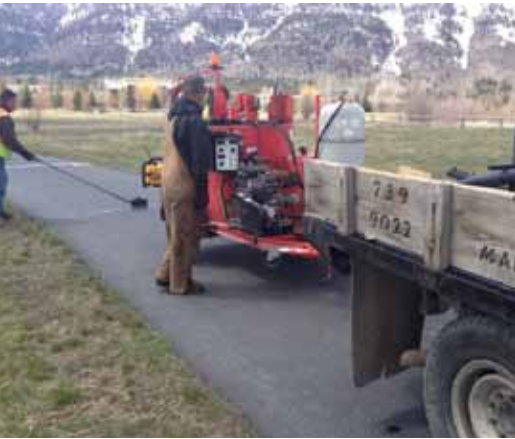
Crack-sealing trail maintenance
