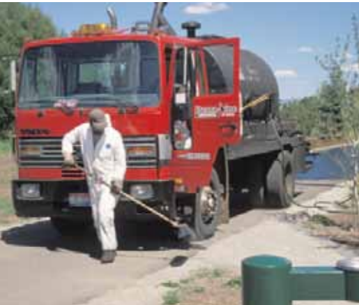
Seal coating trail maintenance
