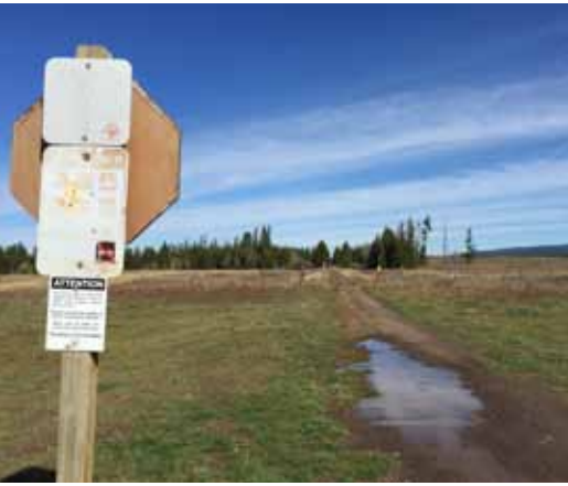
Trail conditions vary considerably along the railroad grade through CTNF. Some portions have held up relatively well while others have experienced rutting and drainage problems.
