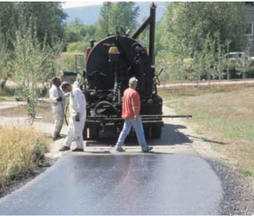
Seal coating trail maintenance
