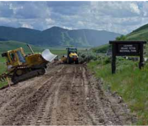
Jackson to Grand Teton National Park pathway construction
