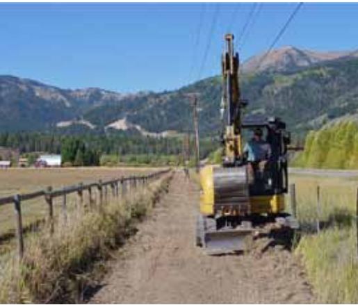
Trail construction along Highway 22 near Jackson, WY
