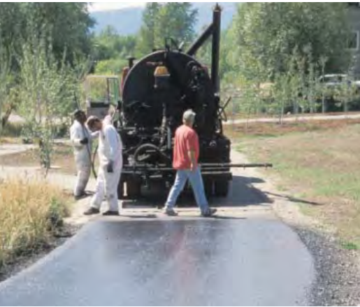
Seal coating trail maintenance
