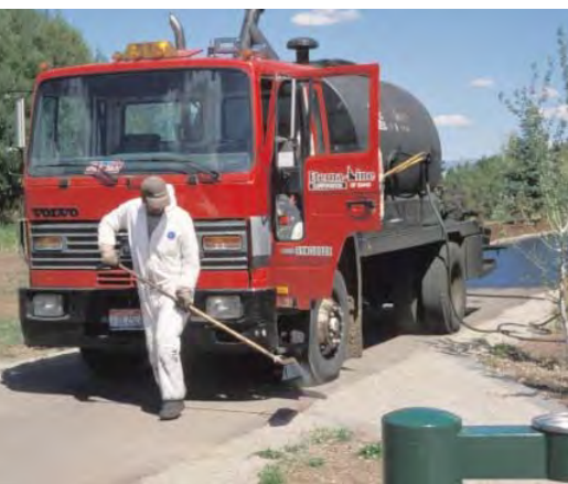
Seal coating trail maintenance
