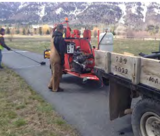
Crack-sealing trail maintenance
