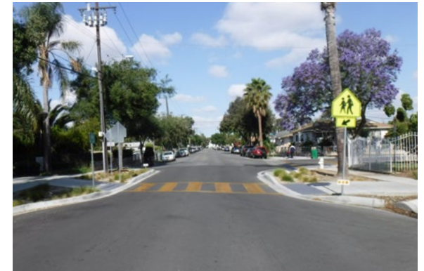
Curb extensions at a school crossing in Santa Ana, CA.
