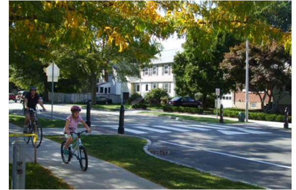
Example of a raised crosswalk.
