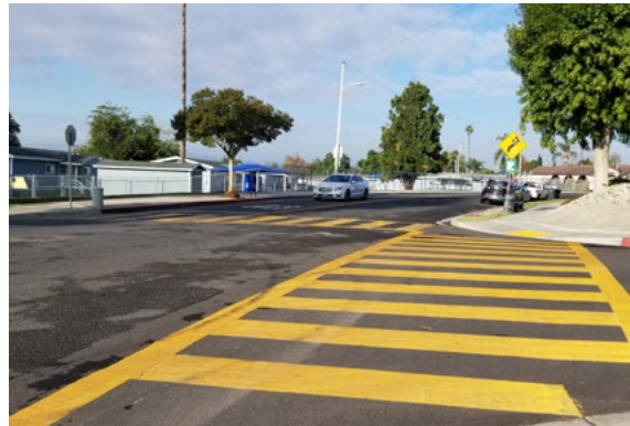
A high-visibility crosswalk outside Hurley Elementary School.
