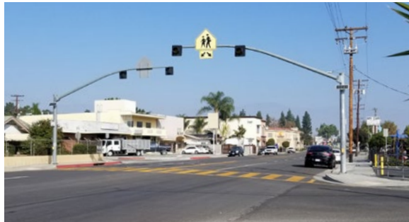
Pedestrian hybrid beacons at a crossing near Sierra Vista Middle School.
