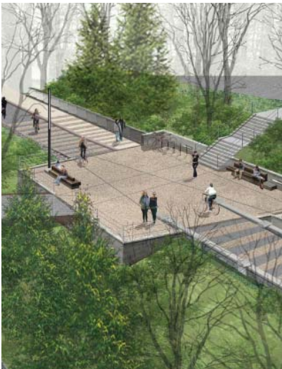
The concept for the Burke Gilman Trail in Seattle, WA includes separating users by mode and creating "mixing zones" at trail intersections.
