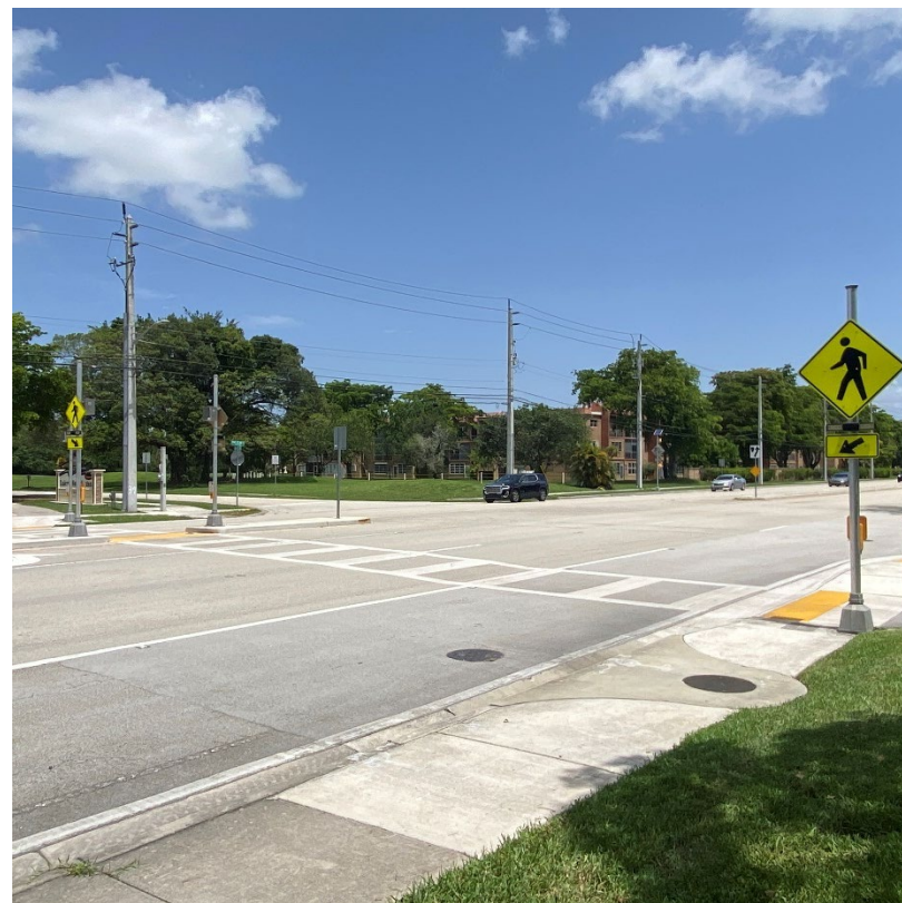
Pedestrian crossing at Colony West Golf Club on N Pine Island Road.
