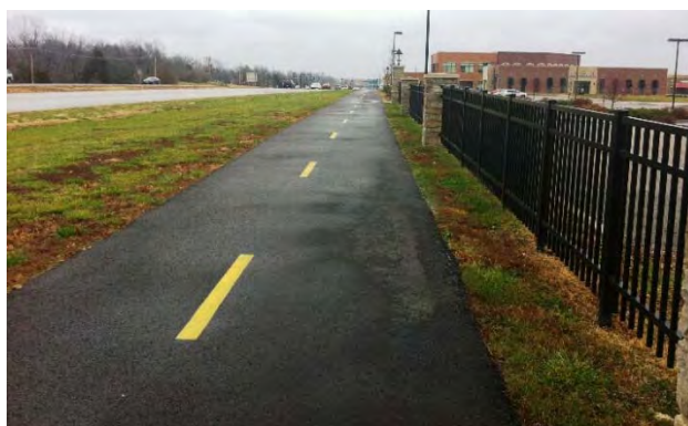
Figure 57: This sidepath incorporates a yellow striped centerline to separate bi-directional traffic.
