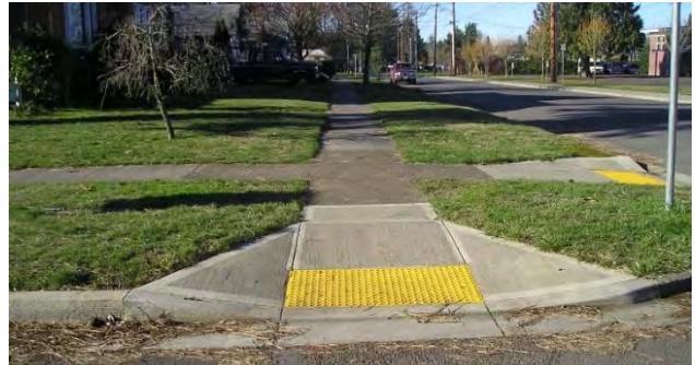
Figure 76: ADA-compliant curb ramps assist persons with physical disabilities in detecting, approaching, and crossing streets.
