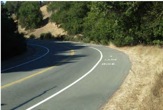
Figure 46: Shoulder bikeways provide a functional facility in rural contexts.
