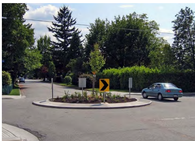
Figure 43: Traffic circles have proven to be effective intersection treatments for bicycle boulevards.
