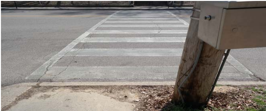
Utility pole blocks a potential curb ramp at the current crossing location
