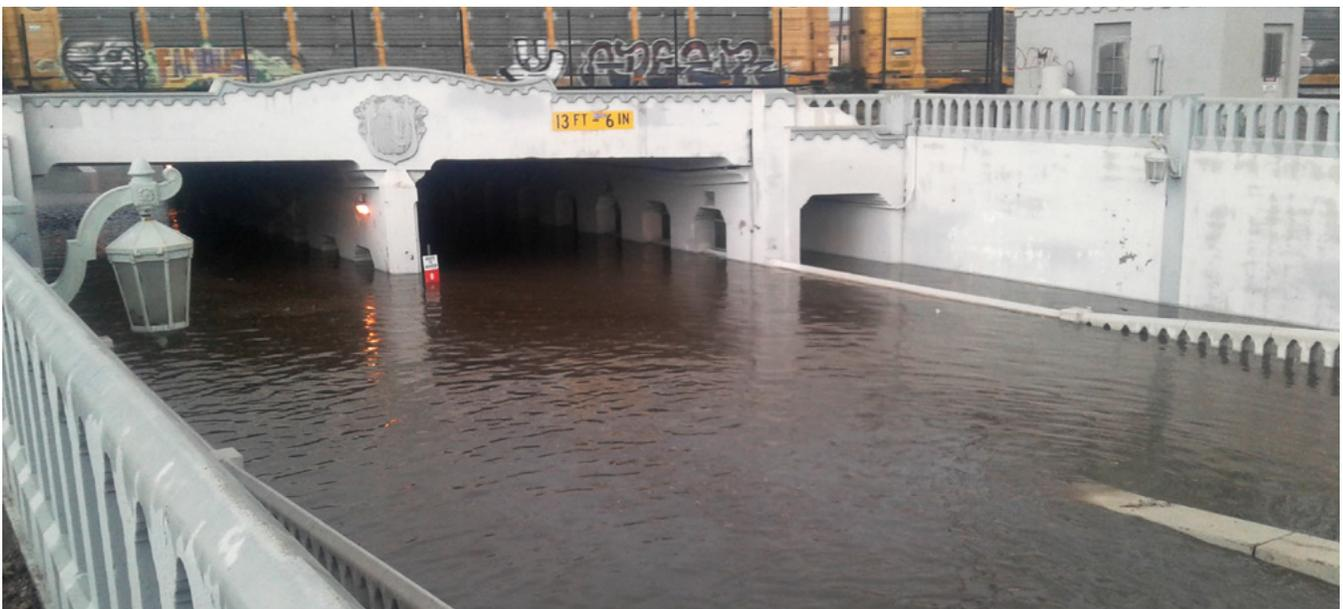
*Limited stormwater infrastructure relies on Tucson's roadways for water conveyance during rain events. In addition to impeding travel during major storms, this also leads to increased pavement maintenance needs.*
