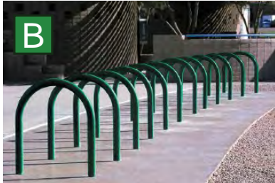
Inverted-U Racks (Type A & B Square on the Bike Rack Placement Map; pg 5-14) provide short term bicycle parking.
