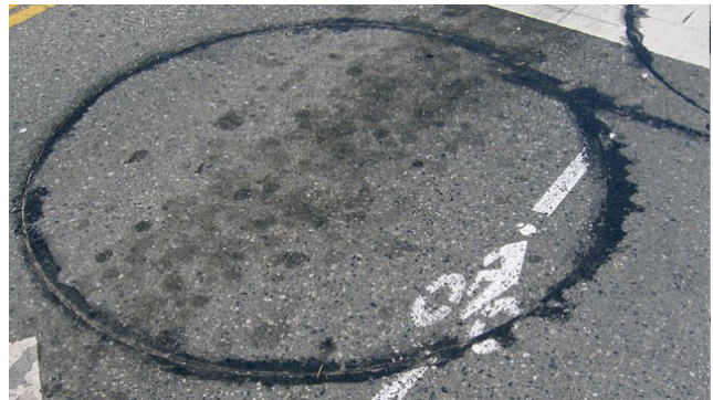
Standard loop detection pavement marking (Photo: NACTO)
