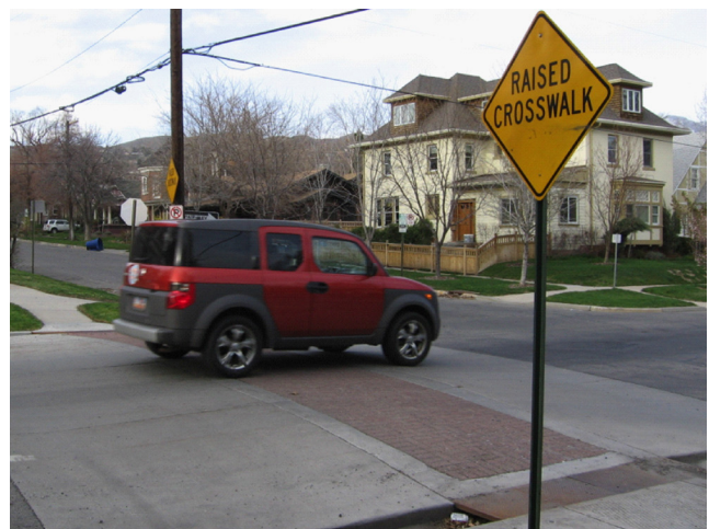
This raised crosswalk on 2nd Ave calms speeds and elevates the crossing for better visibility
