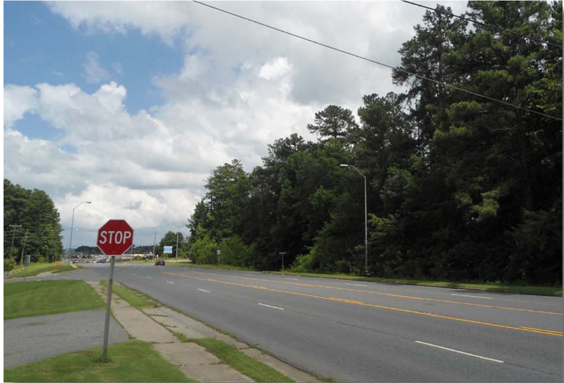
US Highway 64, near the intersection of Pine Glades Avenue
