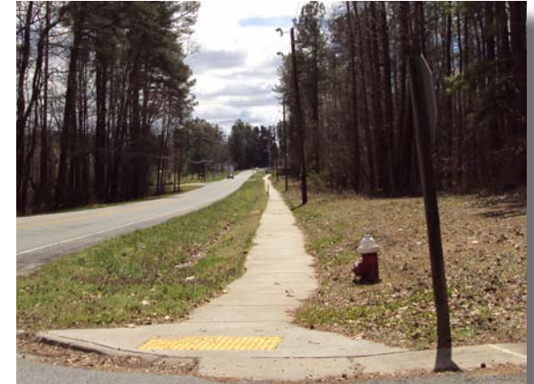
New sidewalk along W. Raleigh Street
