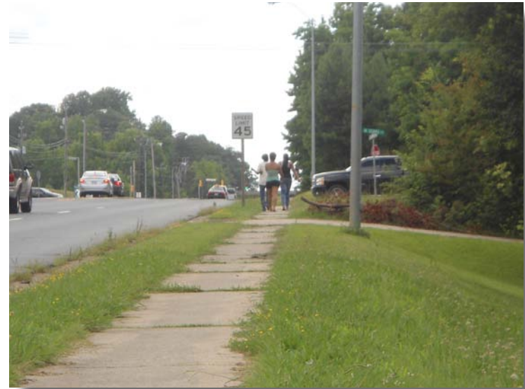
Pedestrians travel on existing sidewalk along the north side of US Highway 64 in Siler City
