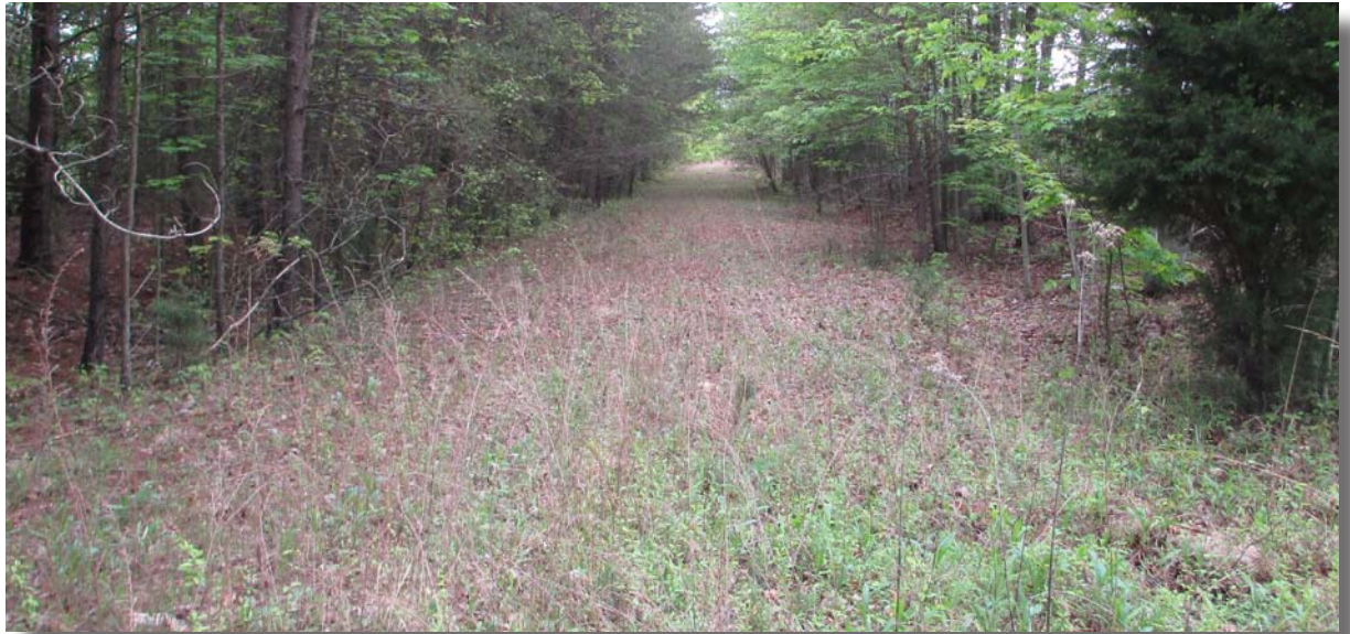
Abandoned rail bed example
