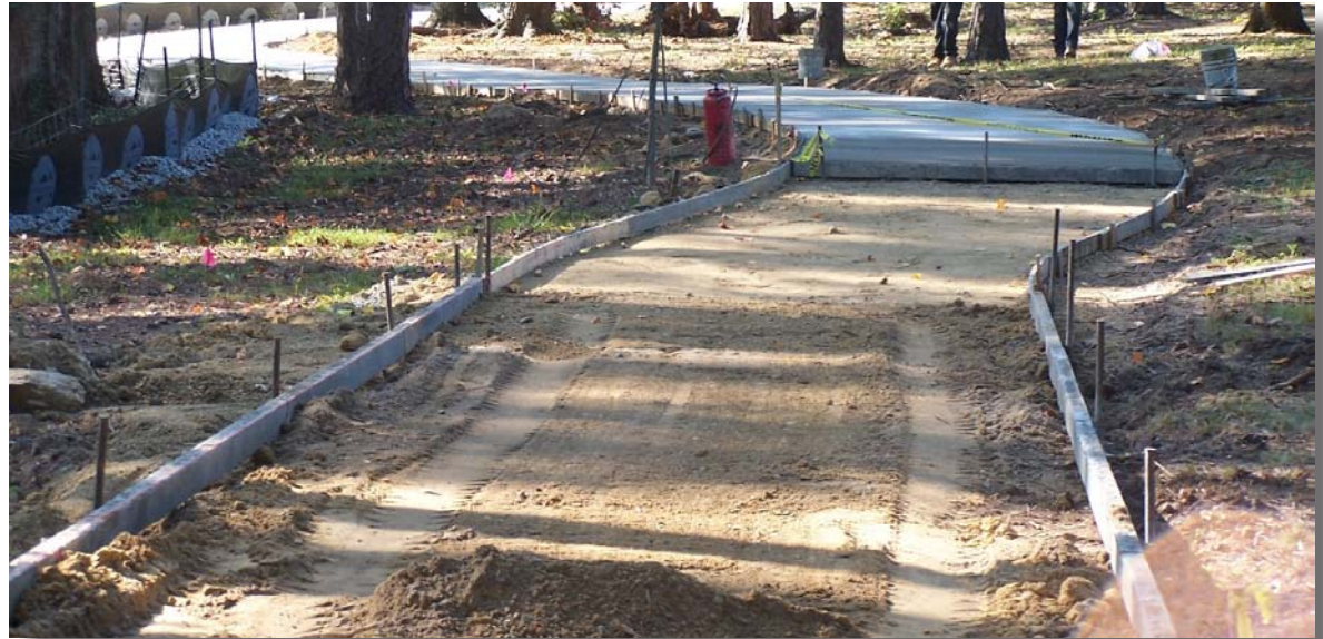
Greenway construction example
