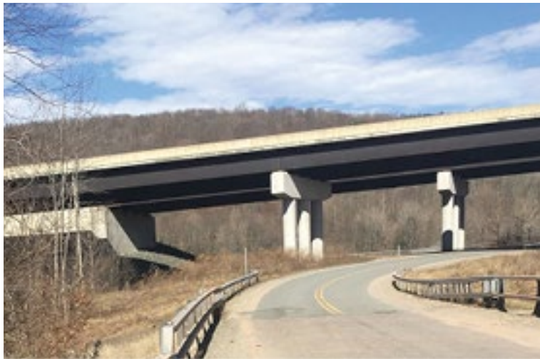
Looking northeast towards the bridge on Fox Mountain Road (BIN 2229030) over the Little Beaver Kill tributary
