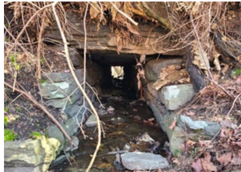
Original O&W stone culvert
