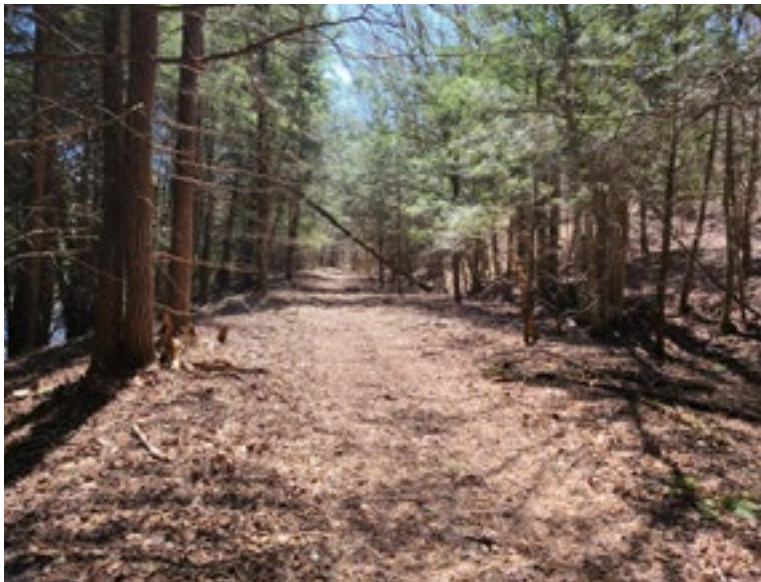
Existing rail bed beyond the washouts is consistent in grade, width, and condition
