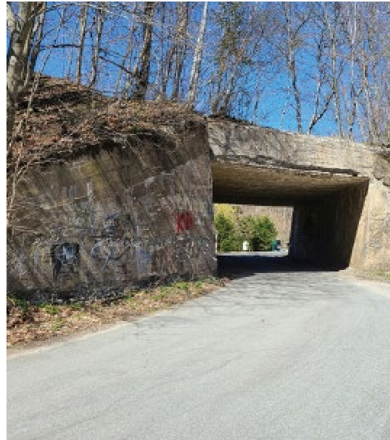
Existing bridge over Old Liberty Road
