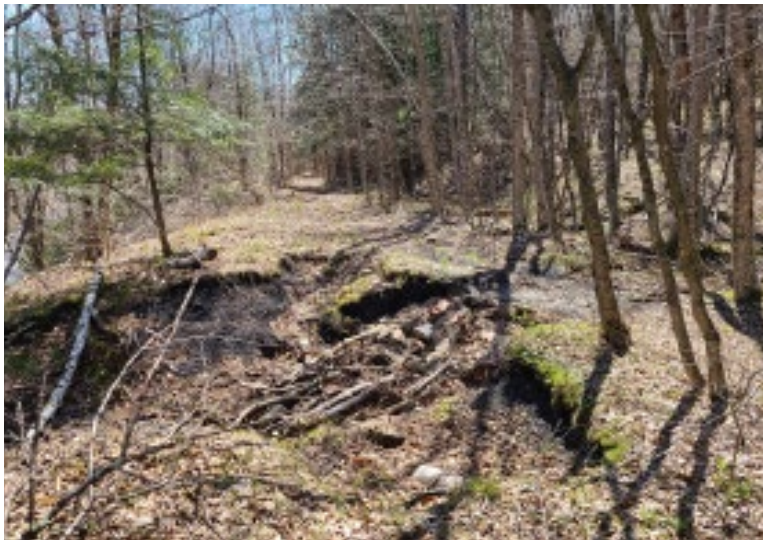
One of the existing washouts that will be addressed with a new closed drainage system.
