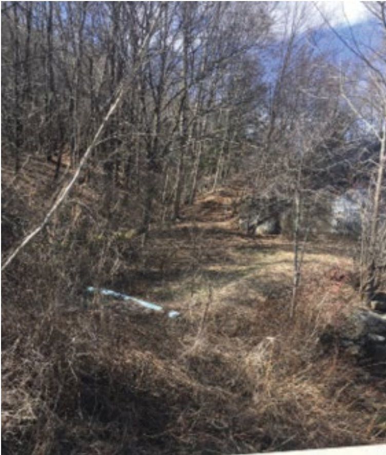
The existing O&W rail bed abutment is still present. A bypass route has been created to traverse to Fox Mountain Road
