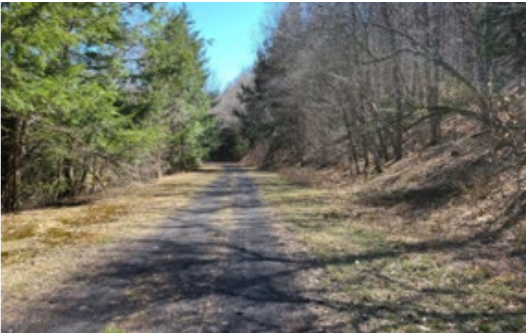
Former vehicular use near the Sonoma Falls attraction has widened the former rail bed corridor
