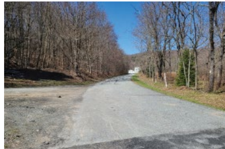
Raveling of the existing pavement is evident due to turnarounds near the Sonoma Falls gate
