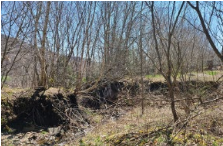
Looking east towards where the rail bed has been washed out. This area to be replaced with a box culvert.
