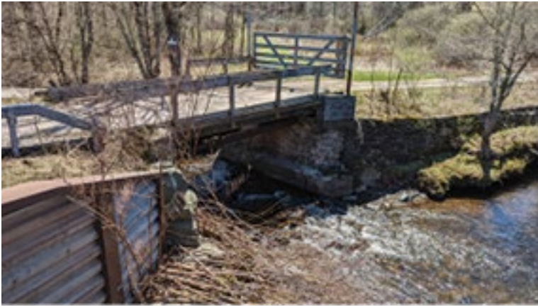
Looking north on Dahlia Road where overhead utility wires would be in direct conflict with the proposed bridge over Dahlia Road
