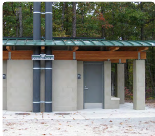
Composting restroom at the current southern end of the American Tobacco Trail in Wake County.
