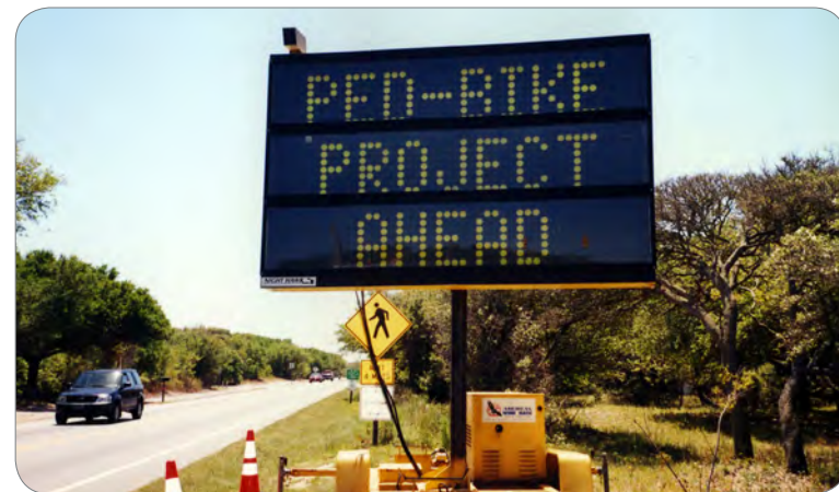
▲ NCDOT Ped/Bike Project Construction.
