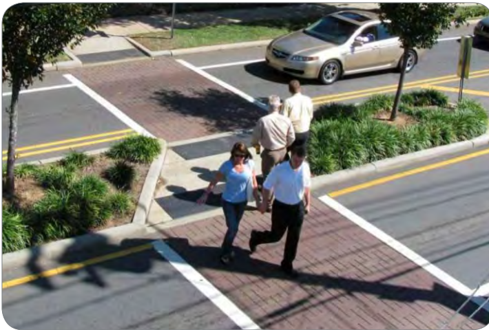
▲ Mid-block crossing construction in Charlotte, NC
