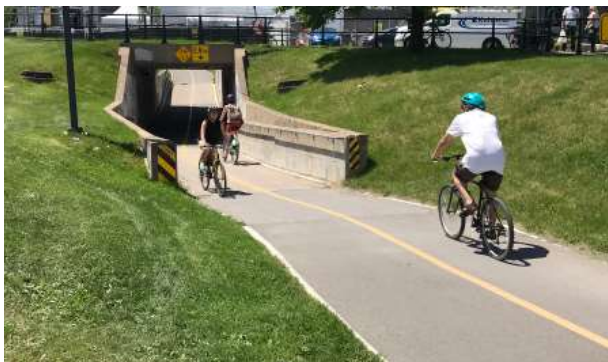
Figure 6.92 – Grade Separated Crossing, Montréal
