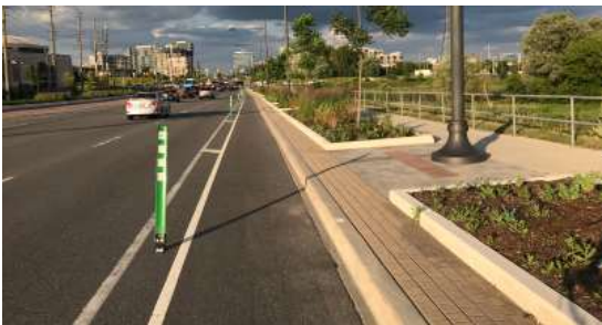
Figure 4.23 – Flex Bollard Separation, Markham
