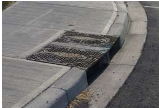
Figure 7.15 – Side-Inlet Catch Basin
