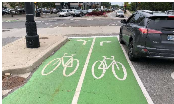
Figure 10.16 – Green Surface Treatment, Hamilton
