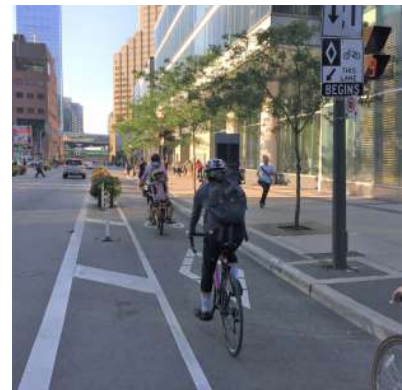
Bicycle Lane Separated by Flex Bollards and Planters, Toronto
