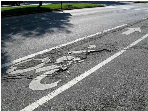
Figure 10.5 – Poorly Maintained Bicycle Lane
