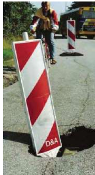
Figure 10.10 – Pothole Identified by Hazard Marker
