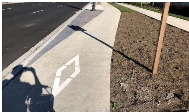
Figure 10.15 – Example of Markings on Concrete (Bicycle Symbol Not Visible)
