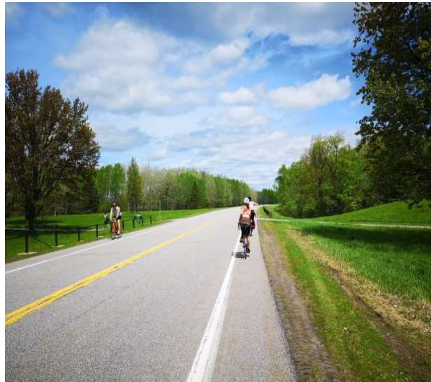
Figure 4.70 – Example of Rural Paved Shoulders, Ottawa
