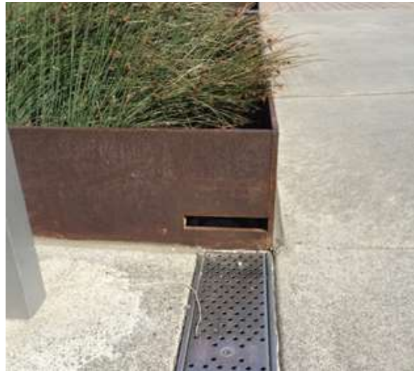
Figure 7.16 – Trench Drain at a Flush Surface
