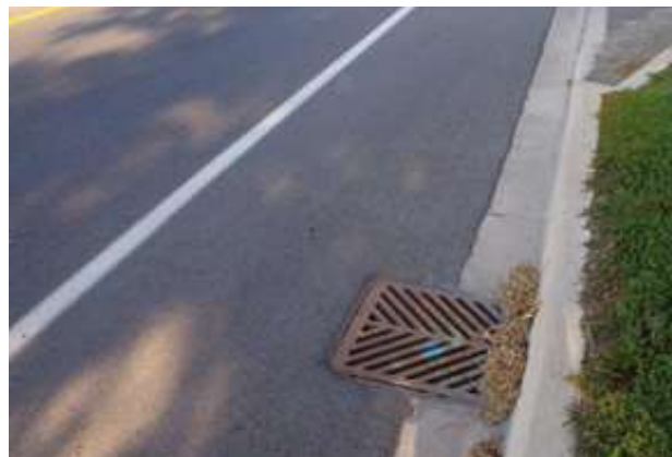
Figure 7.17 – Drainage Grate with Herringbone Openings
