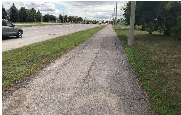
Figure 10.7 – Longitudinal Cracking
