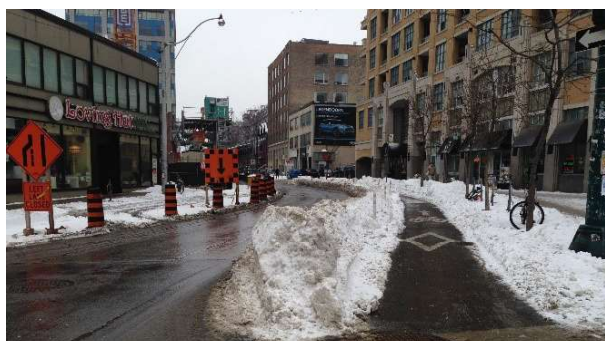
Figure 10.18 – Cycling Facility Cleared of Snow
