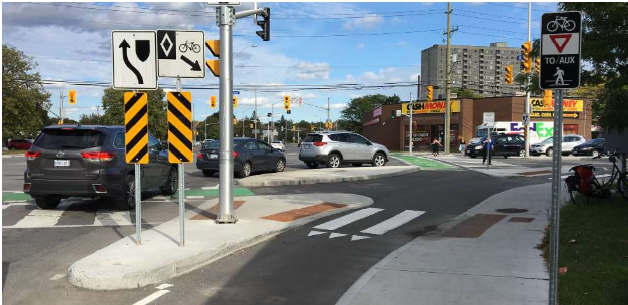
Figure 6.36 – Example of Protected Intersection Corner, Ottawa
