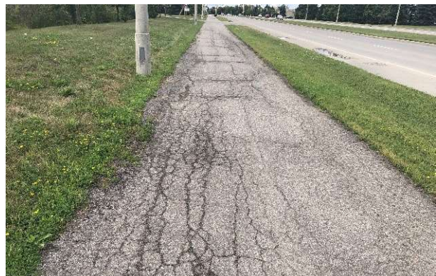
Figure 10.9 – Alligator Cracking
