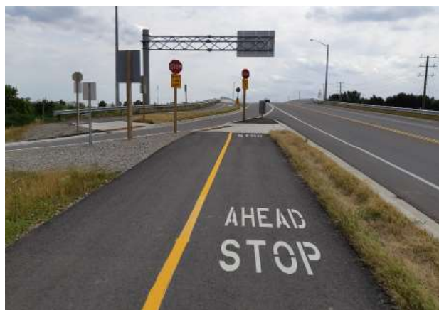
Figure 6.87 – Ramp Crossing, Cambridge
