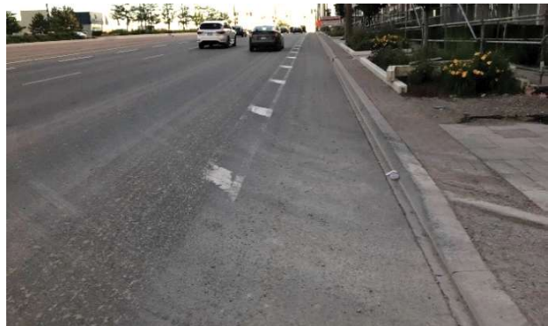
Figure 10.14 – Worn Bicycle Pavement Markings
