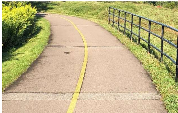
Figure 10.8 – Transverse Cracking
