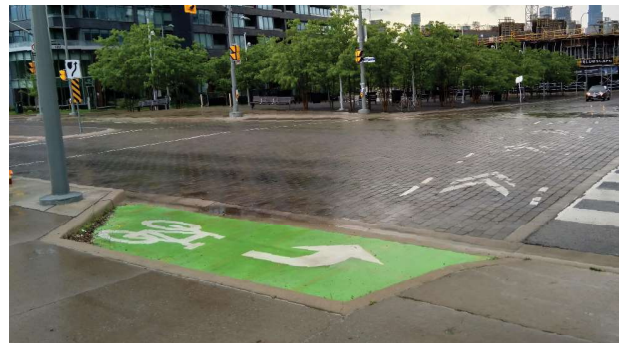
Figure 6.52 – Example of a Pocket at T-Intersection, Toronto
