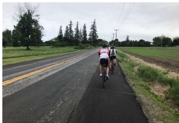
Figure 8.14 – Newly Resurfaced Paved Shoulders, York Region
