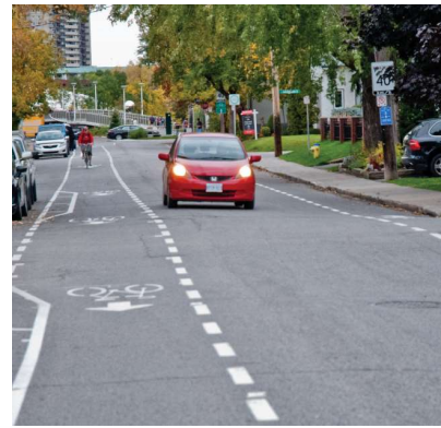
Advisory Bicycle Lane on Urban Street with On-Street Parking, Ottawa
