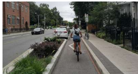
Figure 4.26 – Cast-in-place Concrete Curb Separating a One-way Separated Bicycle Lane, Toronto
