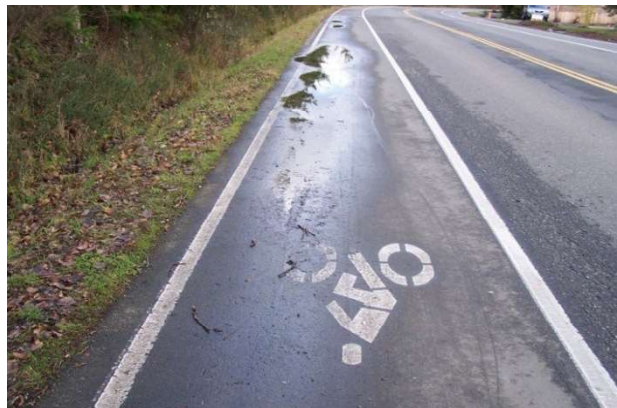
Figure 10.13 – Poor Drainage Causing Ponding in Bike Lane
