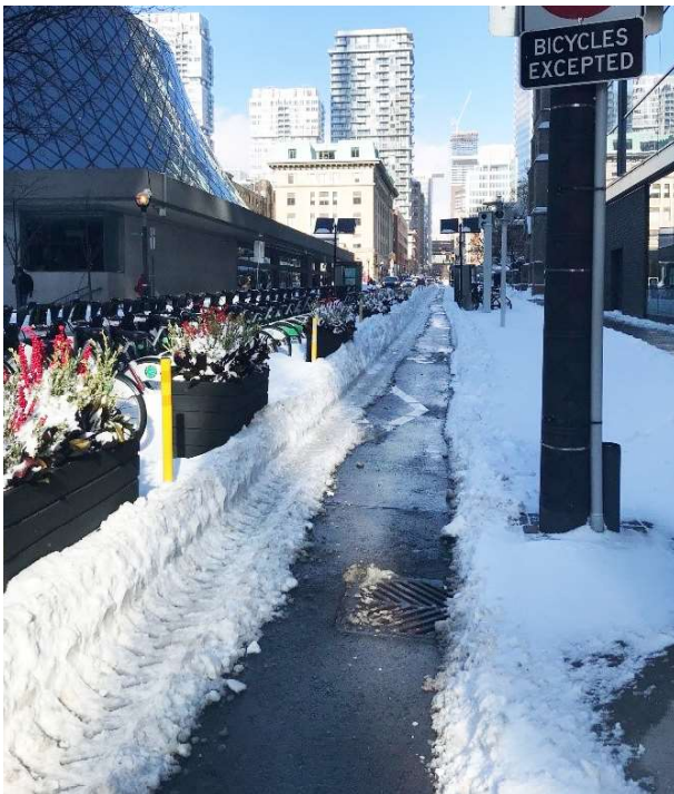
Figure 10.25 – Protected Bike Lane Cleared of Snow, Toronto
